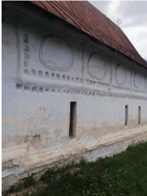
Photo 2: The church in Sălătruc, Argeș (1808)
